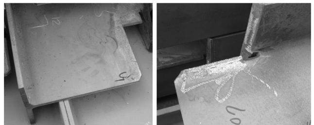
Fig. 7 Wide variety in size and cutting shape of H-beam
