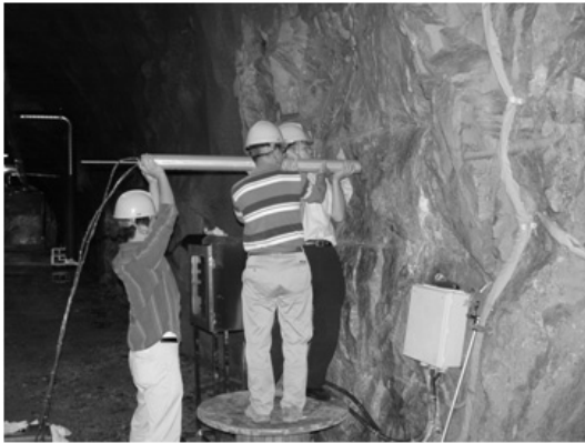
Fig. 5. Installation of the 2 m long heater
