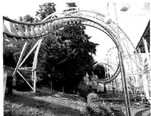
Fig. 8 Roller coaster support structures in Seoul Children's Grand Park
