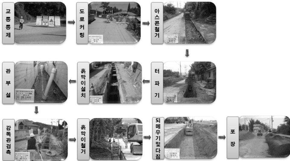
Fig. 2. Construction stages of sewer laying operation.
