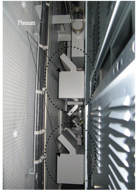
Fig. 12 Installation of the suggested plenum chamber to the TASS console
