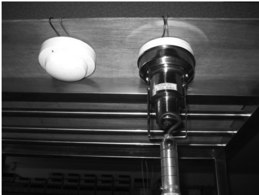
Figure 3. Operating test for heat detector.
