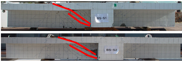
Fig. 8(b) Comparison with failures according to design loads of ledger, when hanger bars anchored in slab of composite beam
