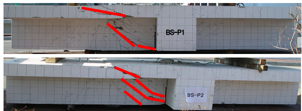
Fig. 9(b) Comparison with failures according to design loads of ledger, when hanger bars anchored in PC web of composite beam
