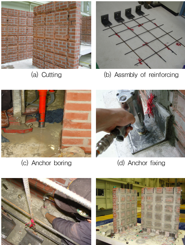
Fig. 7 Reinforcement work for masonry structure
