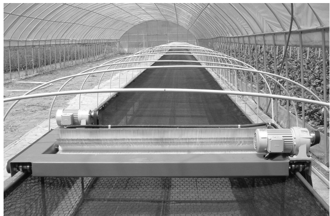
(C) Installation in greenhouse
