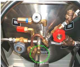
Fig. 1 Fixed tube coupler
