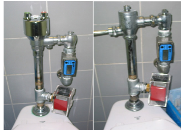
Fig. 4 A water-saving valve and a digital flow meter and the counter device.
