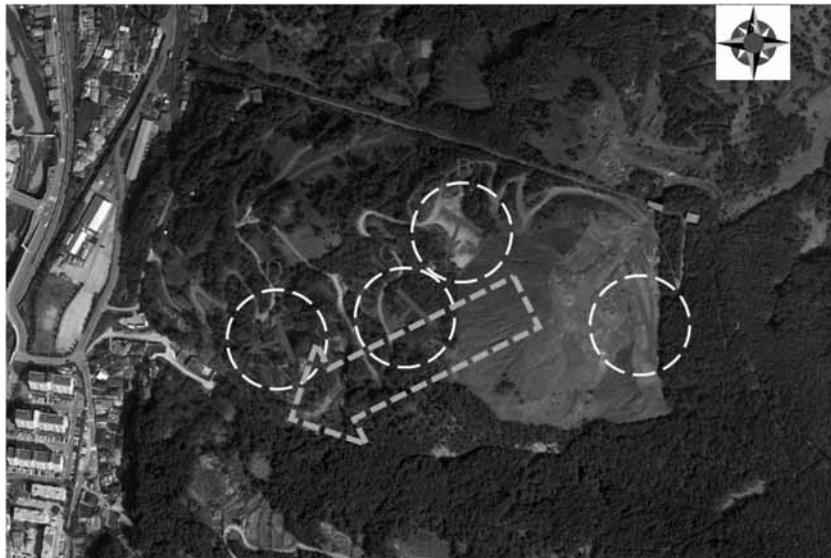
Fig. 22. Direction of ground deformation as determined from the analysis of tension cracks.
