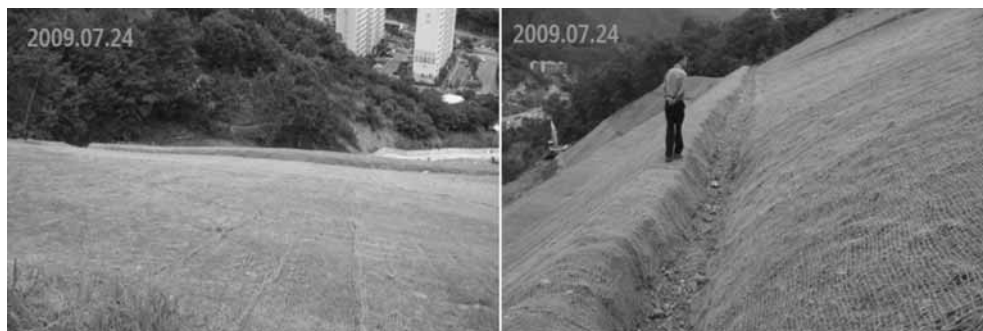
Fig. 19. Completion of cutting work at the lower part of the slope.
