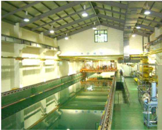
Fig. 1 The facilities of Pusan National University towing tank
