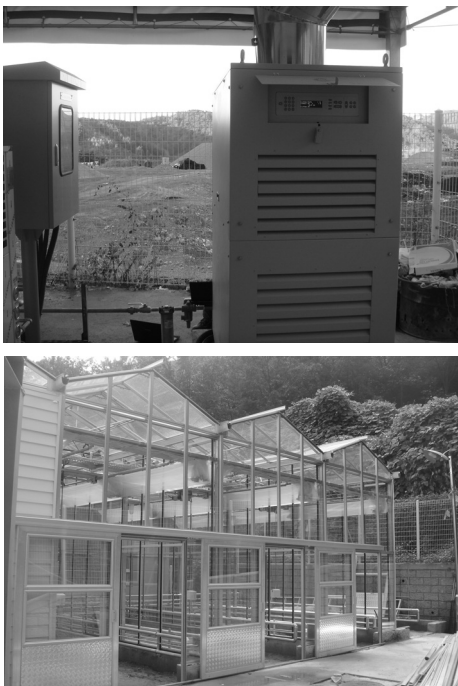
Fig. 5. LFG-MGT power system and green house. (Kwangju-city Land fill site) UP: MGT Output power: 30 kW, 96,000 rpm DOWN: Green house
