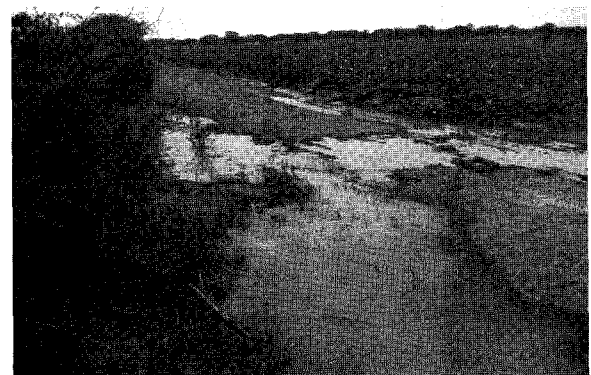
Flattened Existing Canal
