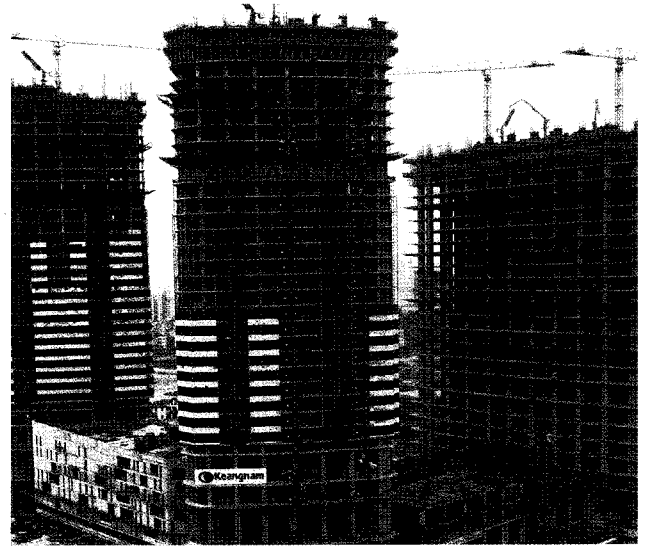
<Hanoi Landmark Tower>
