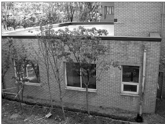
Figure 3. Roof and plastic rainwater facility with concrete manhole for study at 2nd housing complex completed in 2006
