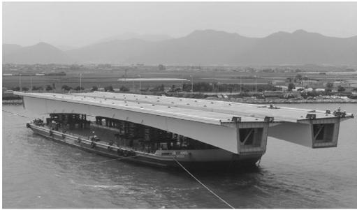
Fig. 2 Pulling of large block with barge
