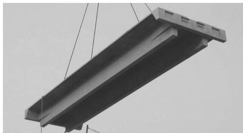
(a) MRS for the one-way joist slab
