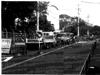
Construction condition of Japan
