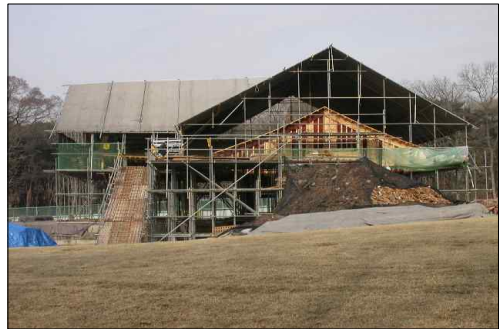
Fig. 2. Jeongjagak, the ceremonial hall in repair
