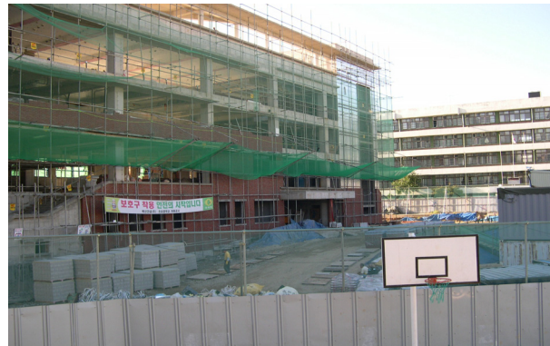
Fig. 6 Front remodeling of school G1.
