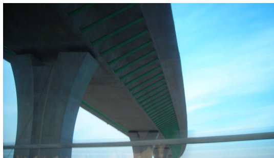
Fig. 1 PSC box girder bridge with RCFFT struts [2].
