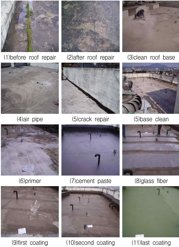
Figure 5. Total construction process
