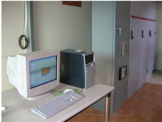
(b) Inverter groups of PV generation.
