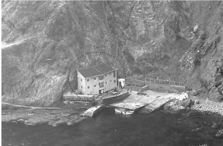
Fig. 11. A bird's eye-view of field installation site
