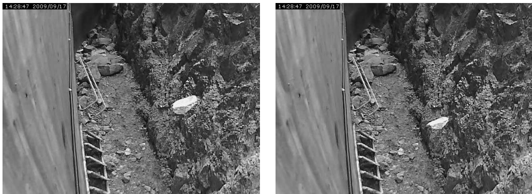
Fig. 14. Captured photos of artificial rock fall experiment at the installation site
