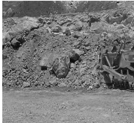
Fig. 7. Improper wall control.
