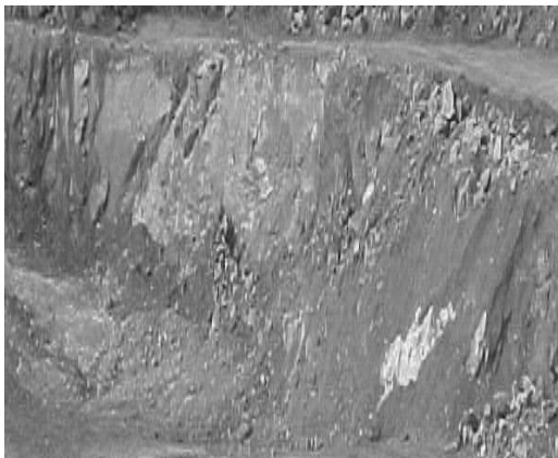
Fig. 18. Almost straight high wall after blast excavation.
