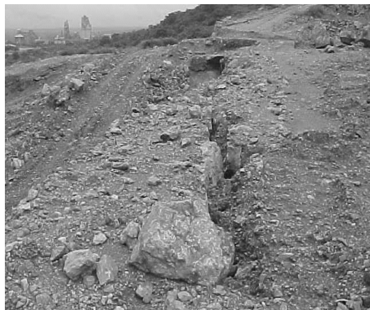
Fig. 5. Severe post-blast back breaking.
