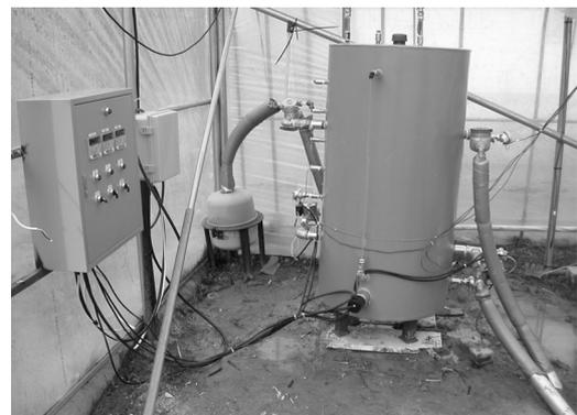
Fig. 2 System of the vacuum type collector and accumulator.
