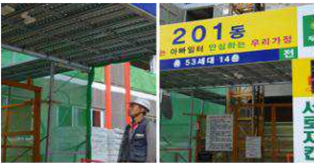
Figure 2. Installation place : Zone B
