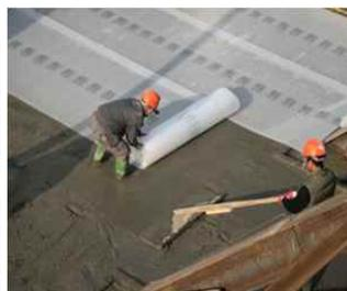
Figure 22. Double layered bubble sheets
