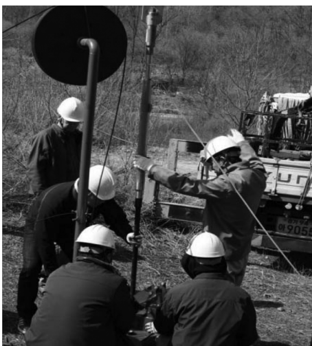
Fig. 4. Field operation of the straddle packer system.
