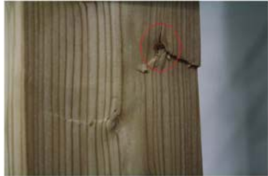
Fig. 3. Failure modes of the compressive specimens (No.1).
