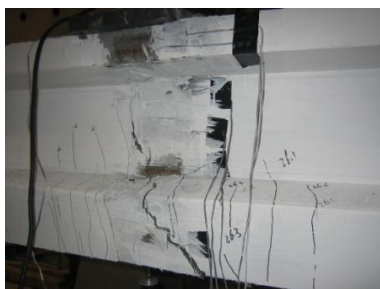
Fig. 20 The state of failure
