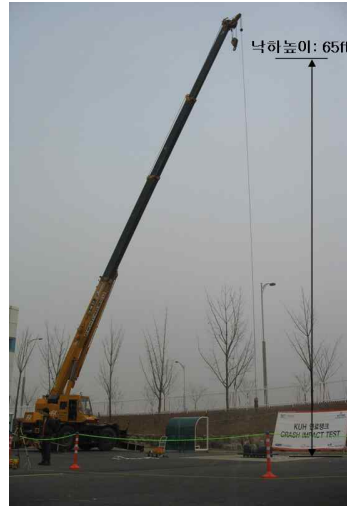
Fig. 5. Site for Crash Impact Test
