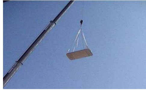
Fig. 9. Step 4 & Step 5: Lifting up to 65 ft and attitude stabilizing
