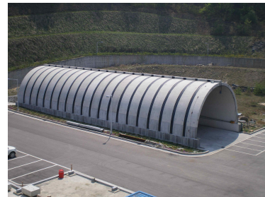
Fig. 2 Photograph of experimental tunnel
