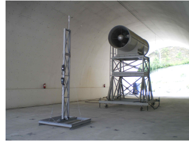
Fig. 1 Photograph of jet fan and velocity measuring apparatus
