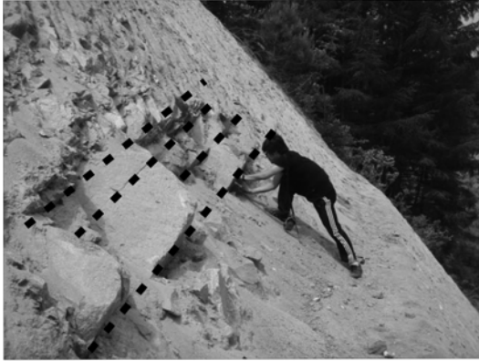
Fig. 8. Status of discontinuities at STA. 0 + 410.
