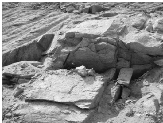
Fig. 4. Rock loss of toe part at STA.0+315.
