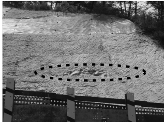
Fig. 7. Exposure at STA.0 + 400~0 + 420.
