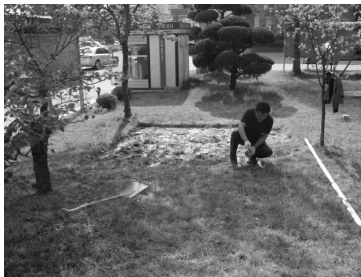
(a) site preparation and grading
