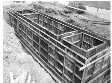
(c) bed erection
