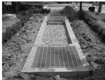
(e) media placement and compaction
