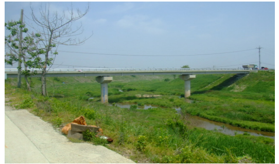
Fig. 4 WPC girder bridge
