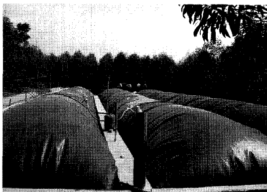
Fig. 1 Biogas HDPE anaerobic digester installed at binh duong province (vietnam).
