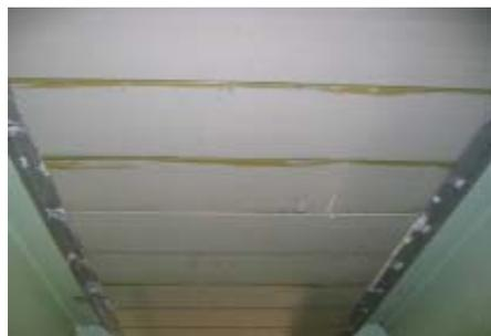
Fig. 5. FRP slab in dunning creek bridge.
