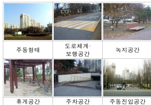
Fig. 6. Asian village apartment construction Photos.
