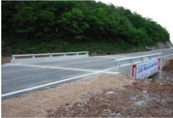
Fig. 9 Completed advanced composites bridge
