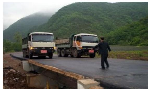
**Fig. 8 Field load testing on completed bridge**
