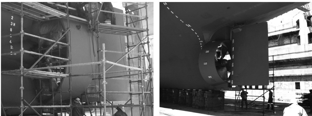
Fig. 1. Installation of nozzle propeller and installed propeller.
