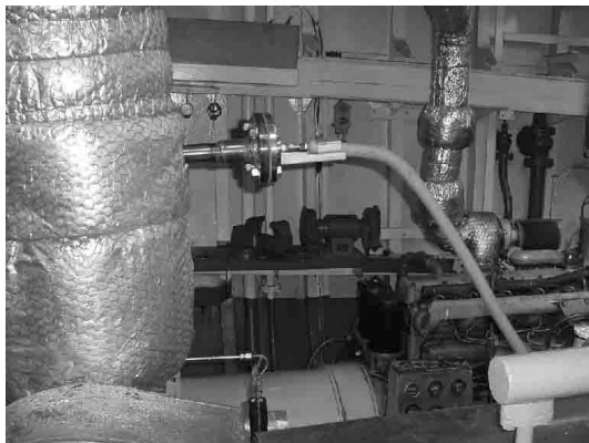
Fig. 5 Installing of probe for NO x analyzer
