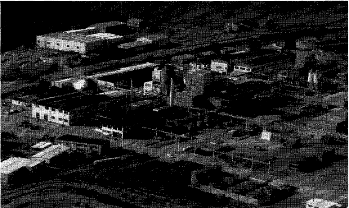
Natural uranium to UF 4 conversion plant, Comurhex Malvesi, France
