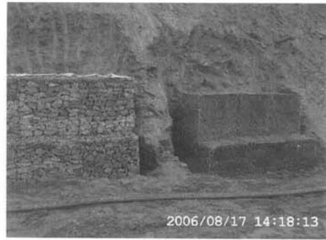
Figure 3. Steel framed retaining wall, existing gabion retaining wall and new gabion retaining wall with vegetation base materials.
