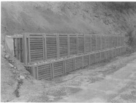
Figure 3. Steel framed retaining wall, existing gabion retaining wall and new gabion retaining wall with vegetation base materials.
