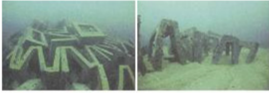
Fig. 4 Artificial reefs deployed at samcheok coastal waters in Korea (Artificial reefs were installed at a depth of 1~12 m)
