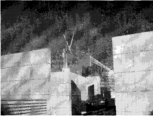
Fig. 1. Vertical wind turbine installed on top of a building.
