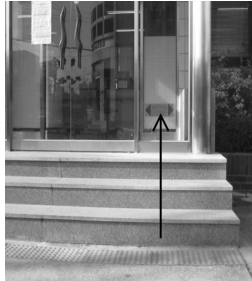
Fig. 2 A field investigation of inundated depth during the flooding at Samcheok City
