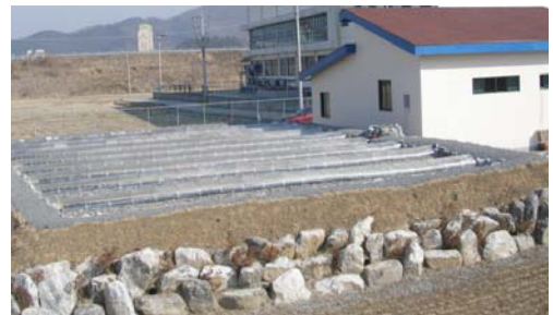
Fig. 2. Photograph of the bio-industry wastewater treatment plant.
